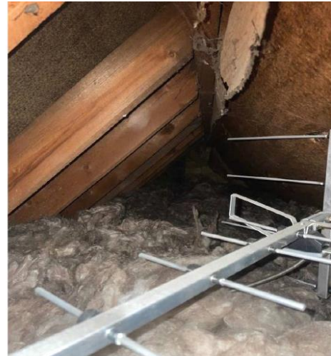
MI Roll fitted to horizontal roof space
